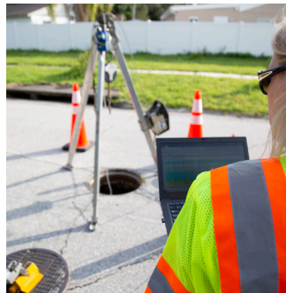
Hillsborough flow monitoring
